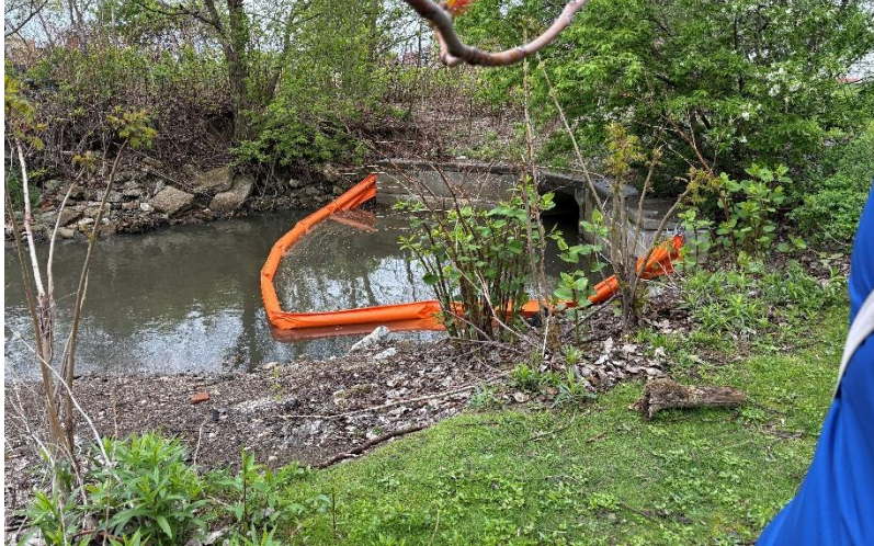
Litter boom installed on Erie Water Works property.
