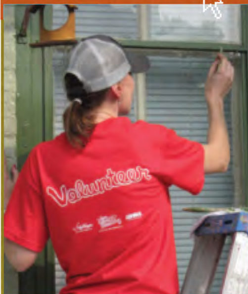
Fresh Paint Days West Reading, Berks County
